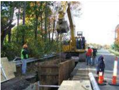
Figure 10.3-8 Onshore Open Trench and Duct Bank
