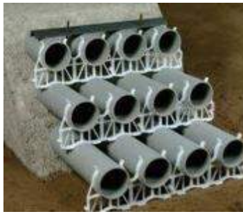
Figure 10.3-8 Onshore Open Trench and Duct Bank
